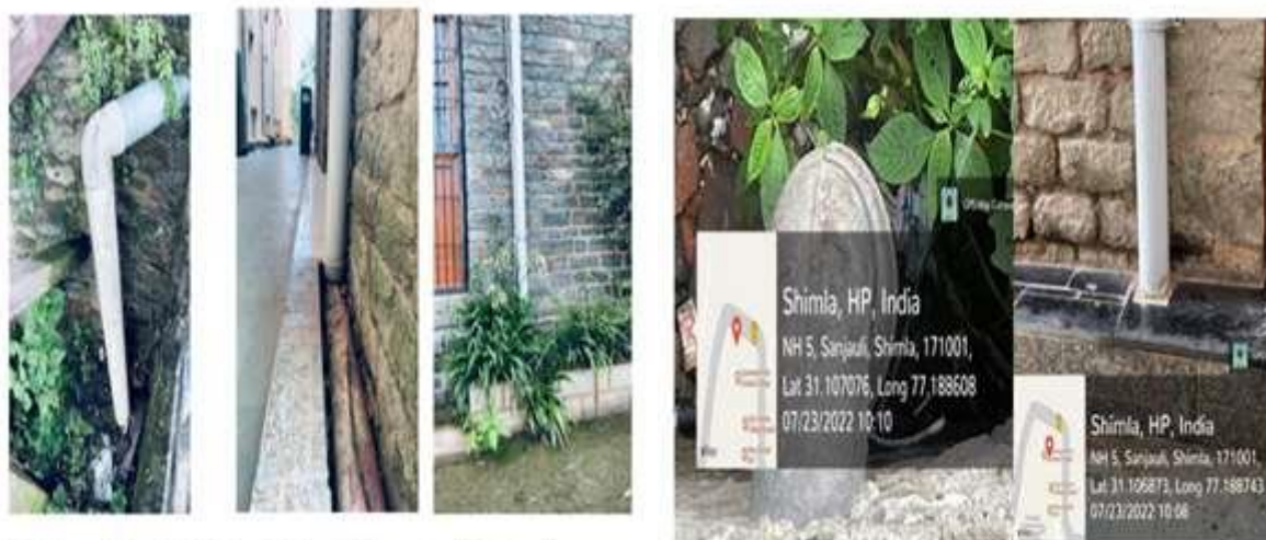
PVC pipes used to reach the rain water to the tank from various buildings' roof
