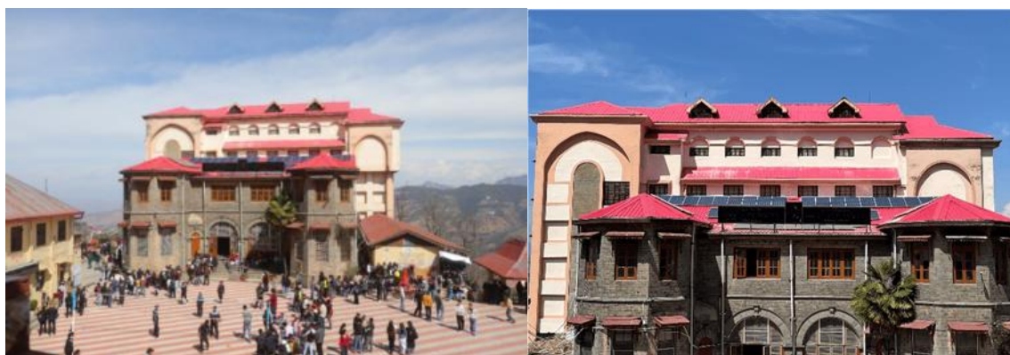
Solar panels installed on the campus building.
