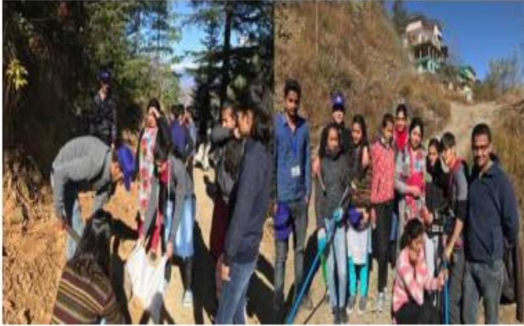
NSS VOLUNTEERS AT ADOPTED VILLAGE KUFUR NEAR BHRARI MAKING AMBULANCE ROAD ON 21ST DECEMBER 2017
